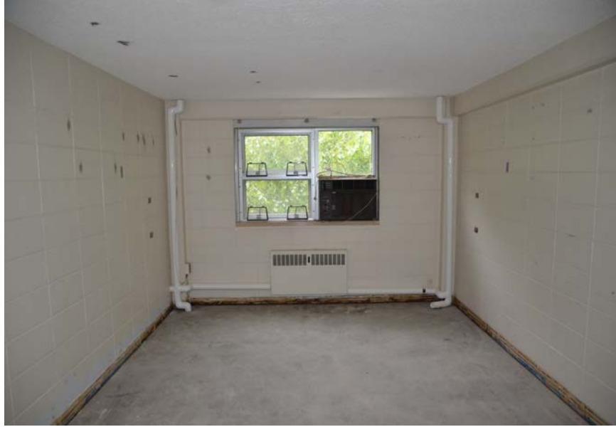
Typical Guest Housing Room (Exterior Wall)
