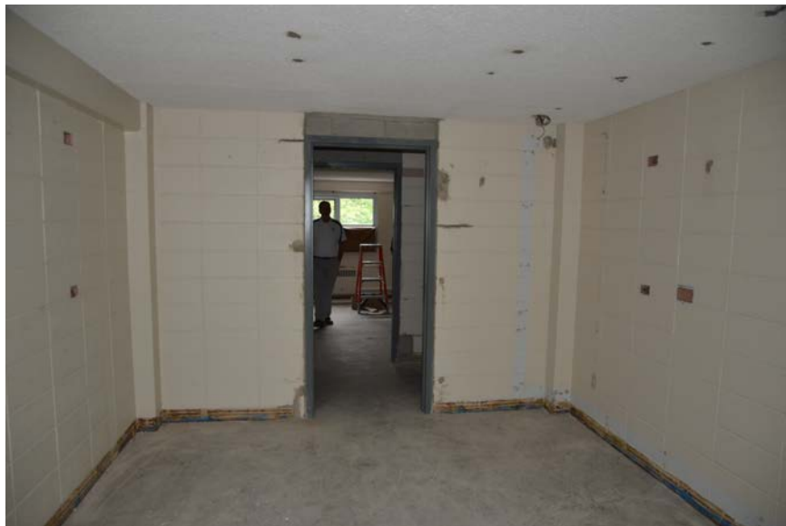
Typical Guest Housing Room (Interior Wall)
