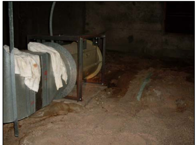
Crawl Space Ventilation
