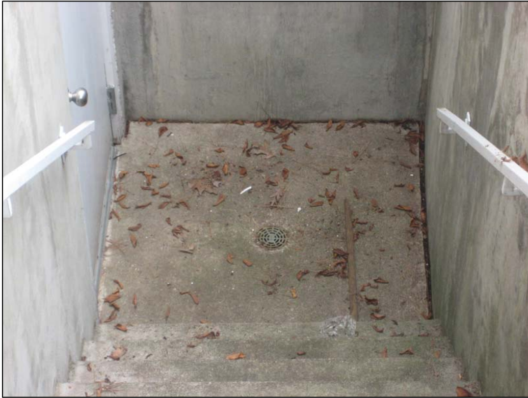
Drain at Bottom of Basement Exit Stair
