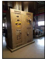
MAIN SWITCHBOARD NO SCALE
