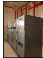
12.47KV SWITCHGEAR NO SCALE
