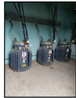
VAULT TRANSFORMERS NO SCALE
