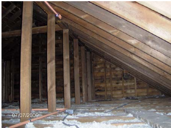
Image 6: Rafter and ceiling joist framing in roof
