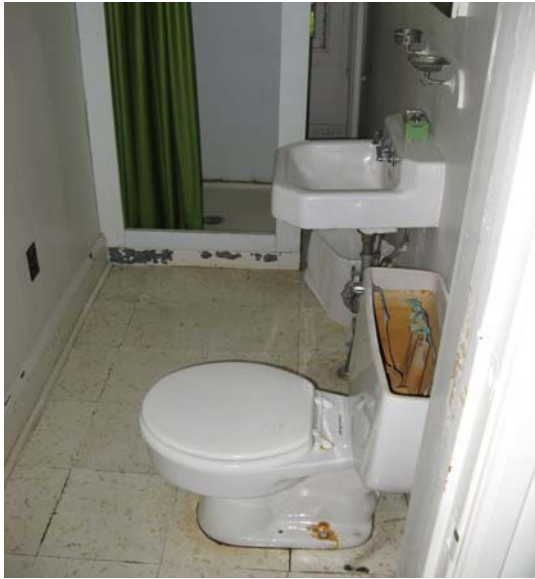
Image 13: Bathroom shows peeling tiles, incomplete fixtures, and changes made over time (note relatively modern toilet).
