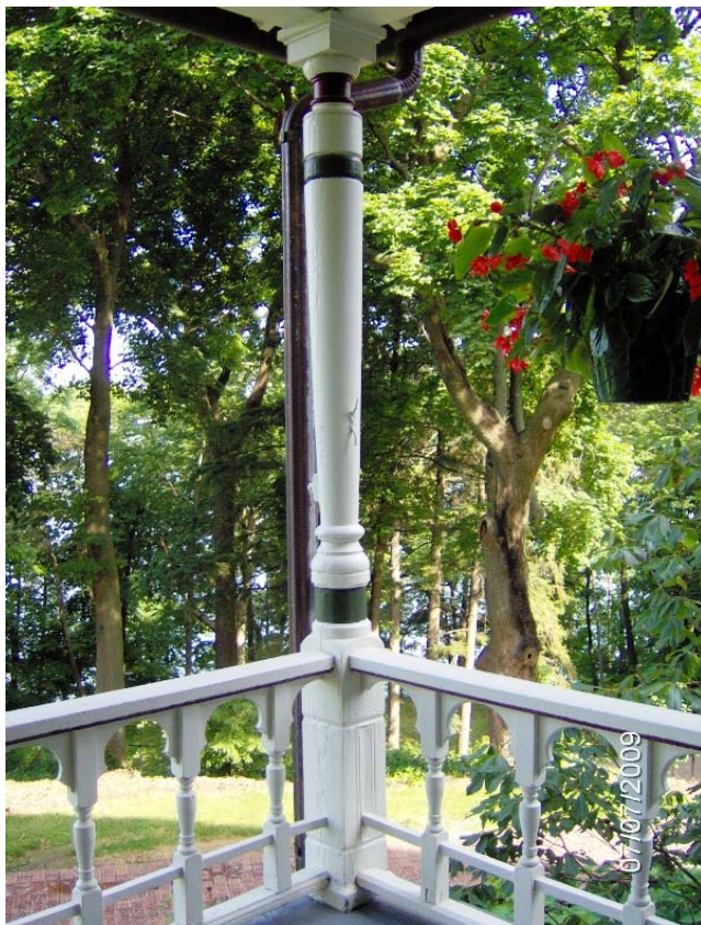
Image 11: Typical porch column
