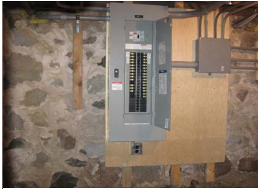
New service panel installed in the basement in 2006
