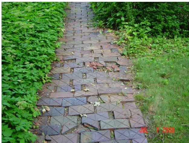
This close-up of a walkway reveals bricks that are crumbling and uneven
