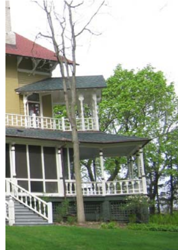
Current picture shows the widened first floor porch (see noted plan diagram pg. 51)
