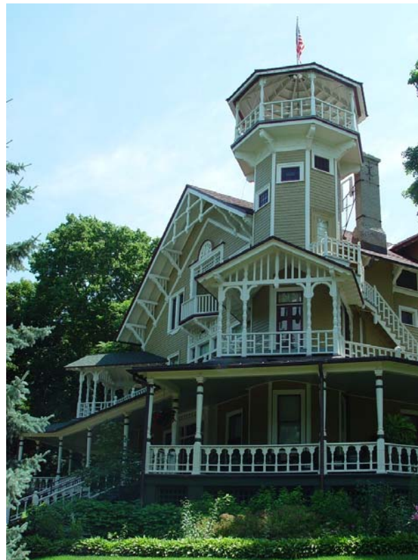
View showing the four-story tower on the northwest corner of the house. Much of the “stick work” is visible, including eave brackets, posts, railings, spindles and angle braces.
