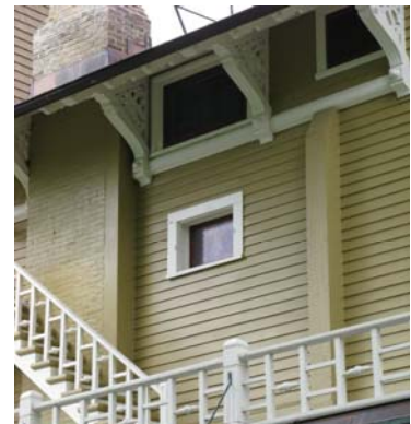
Plumbing chases were added to the exterior (various dates)
