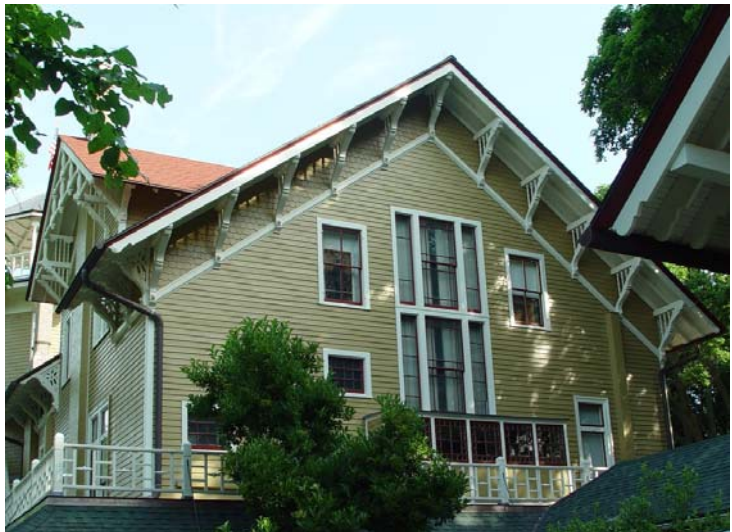
The south elevation has some unique features, including a large window wall in the main staircase, and an absence of the large gable brace found on the other elevations
