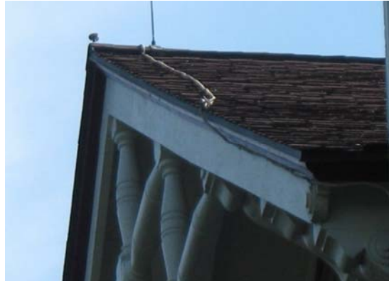
The existing lightning protection system was inspected and repaired in 2006
