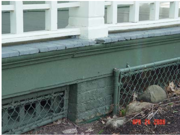
Images 7: Original lattice work is covered by chain link fence
