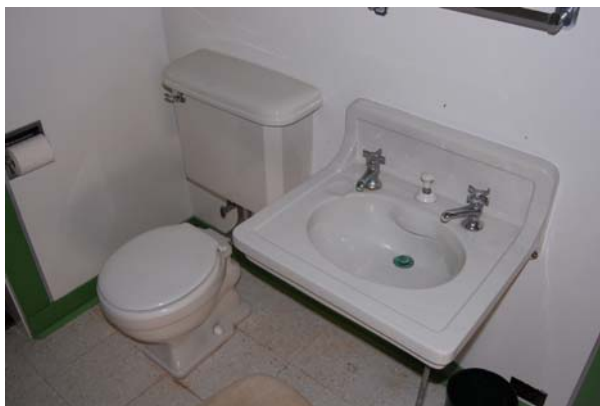
Typical bathroom fixture thought to be dated early 1900's
