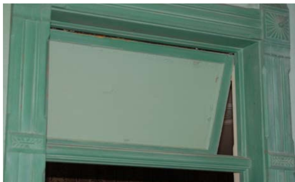
Typical transom window above an interior door
