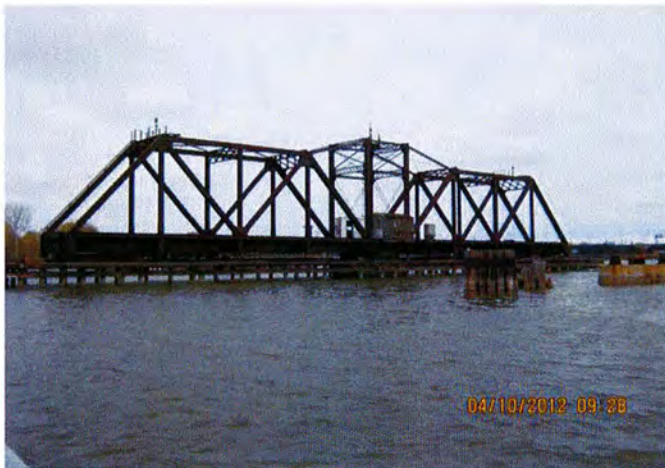
Porlier Street Bridge, Green Bay, WI (East side view)
