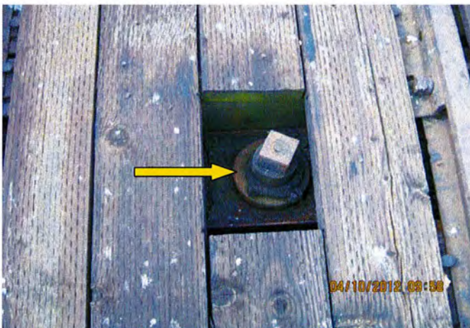
Asbestos Sample 05, rope gasket center of bridge
