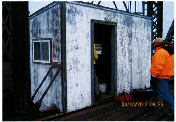
Small wood shed on west side, assumed ACM roofing
