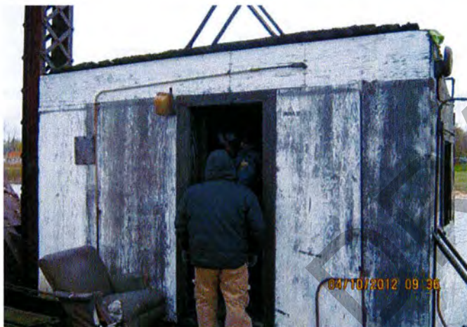
Small wood shed on east side, assumed ACM roofing
