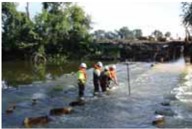
Southern Access Stage II
