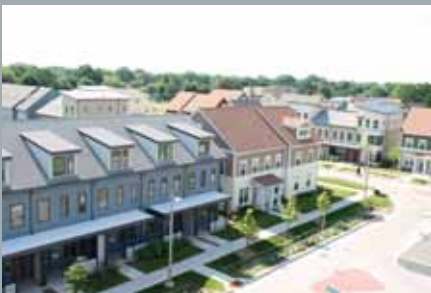
Westlawn Gardens Housing Revitalization Milwaukee, WI
