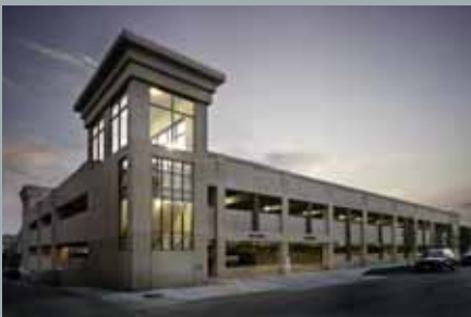
Parker Drive Parking Structure Janesville, WI
