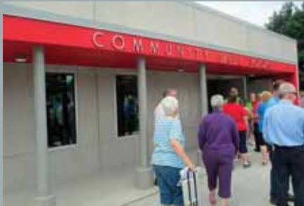
Highland Manor Community Safe Room Madison, WI
