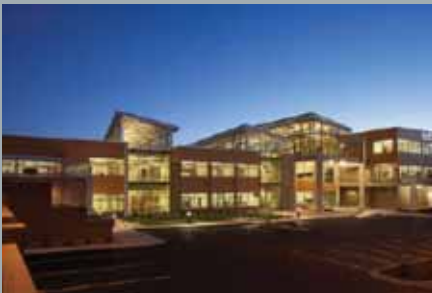
Tri-North Builders Headquarters Madison, WI
