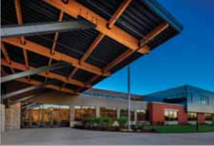
Williams Bay Elementary School Williams Bay, WI
