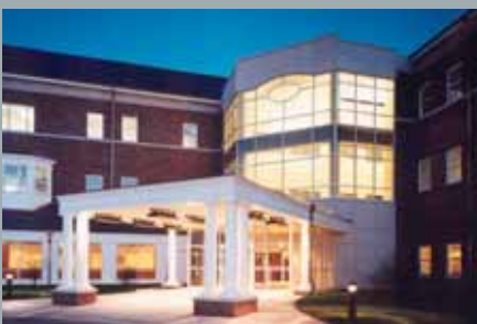
Lake Forest Hospital Medical Office Bldg. Grayslake, IL
